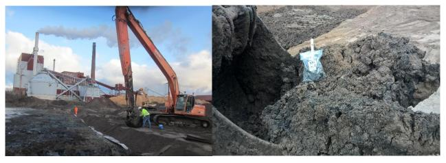
Figure 7. Sampling for technical testing during stabilization works.
