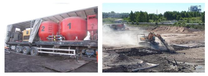
Figure 12. Dry binders were mixed on site by blowing them in different tanks several times before the mass stabilization. Two different binder mixtures (e.g. fly ash and cement) can be fed at the same time to the excavator with mass stabilization equipment.
