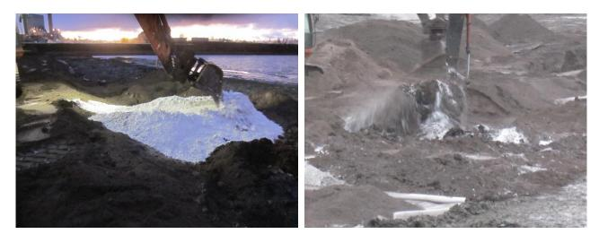
Figure 5. Spreading and premixing of gypsum waste to sediment with excavator.
