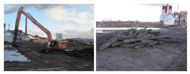
Figure 4. Removal of logs from the basin before mass stabilization carried out by excavator with attached rake head
